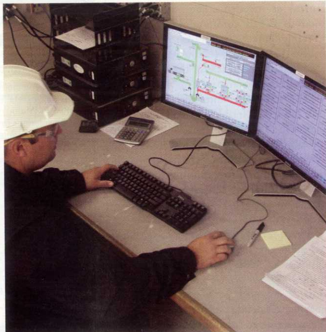
BCI Project Manager Adam Hinton checks on the system in the GTEC control room. For more photos, see this article under www.control.com/archives . Source: Bachelor Controls
